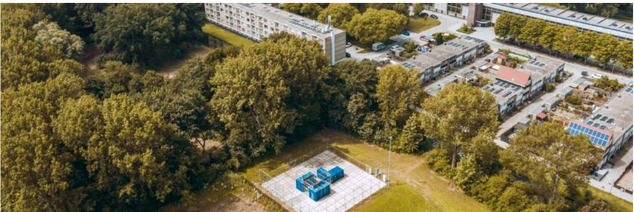
Figure 14: Local hydrogen heat for residential buildings in Rozenburg, Netherlands
